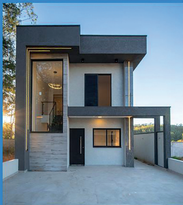
COND. VILA TOSCANA - CAJAMAR
